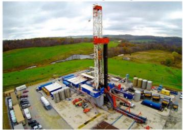
Drilling rig must leave location prior to frac operations
